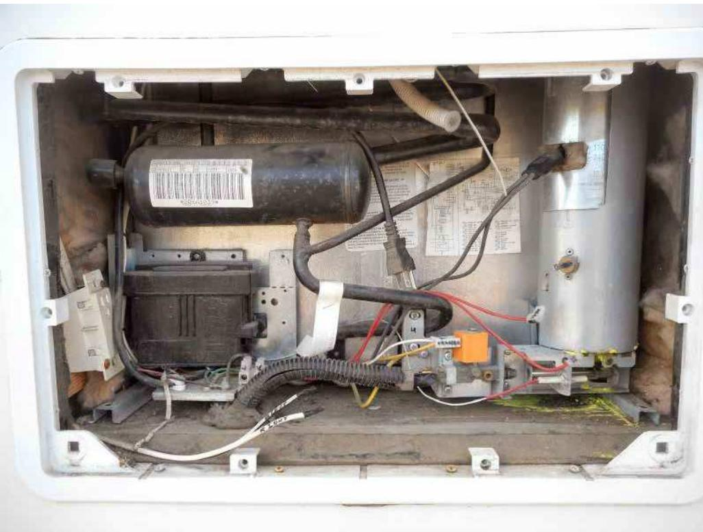
The back of a fridge can be a complex place, especially in a three-way unit like this. Clean carefully to maximise airflow and inspect wiring and any gas fittings to ensure all are in good condition.
